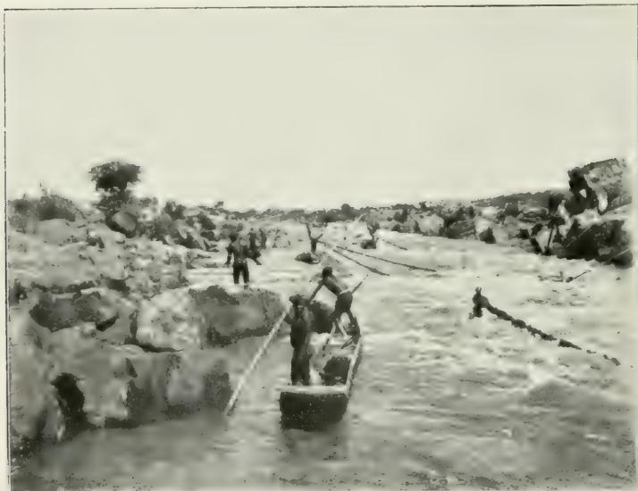
Photo by Capt. C. H. Foulkes, R.E.
